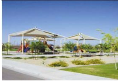
Pyramid Mast Panel Structure
