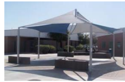
Hexagon Mast Panel Structure
