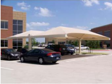
Full Cantilever Double Wide Structure
