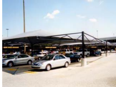
Tri-Truss Double Wide Structure
