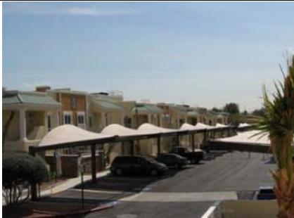
Single Center Bow Structure
